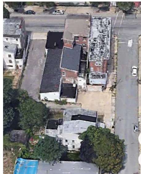
Rear Overhead View
