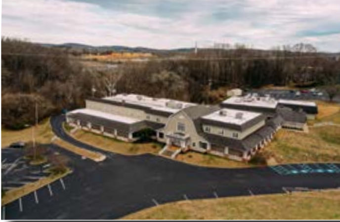
Kinser/Admin. Building: 37,365 SF | 1989 | 2020
