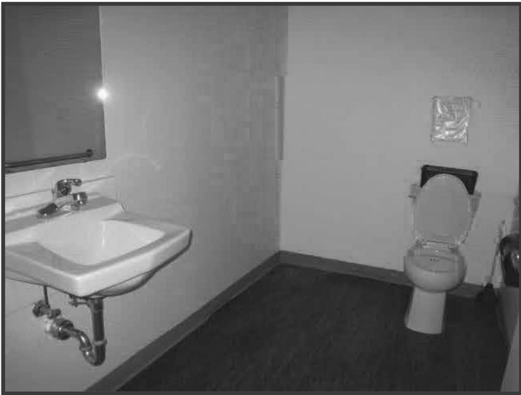
INTERIOR VIEW OF BUILDING
