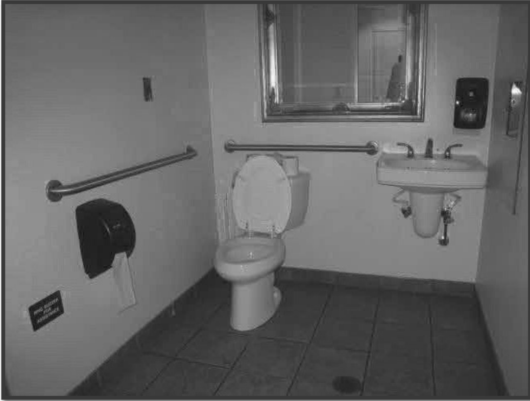
INTERIOR VIEW OF BUILDING
