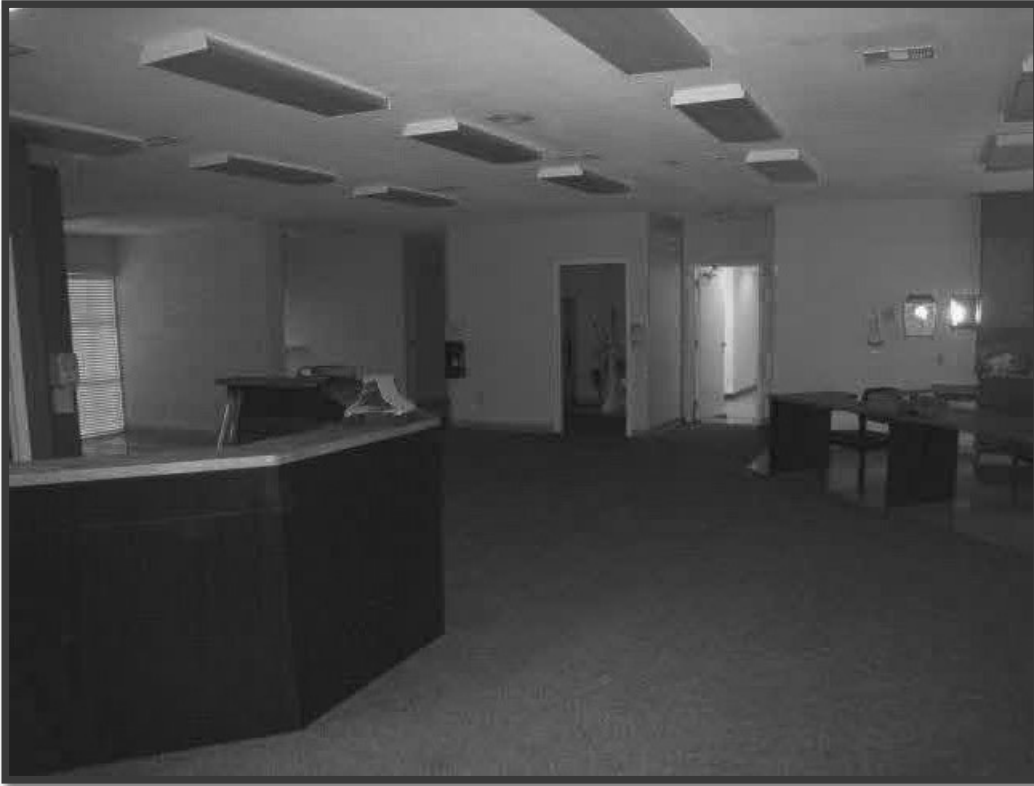
INTERIOR VIEW OF BUILDING
