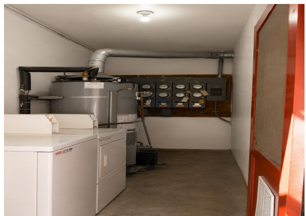
Laundry & Utility Room
