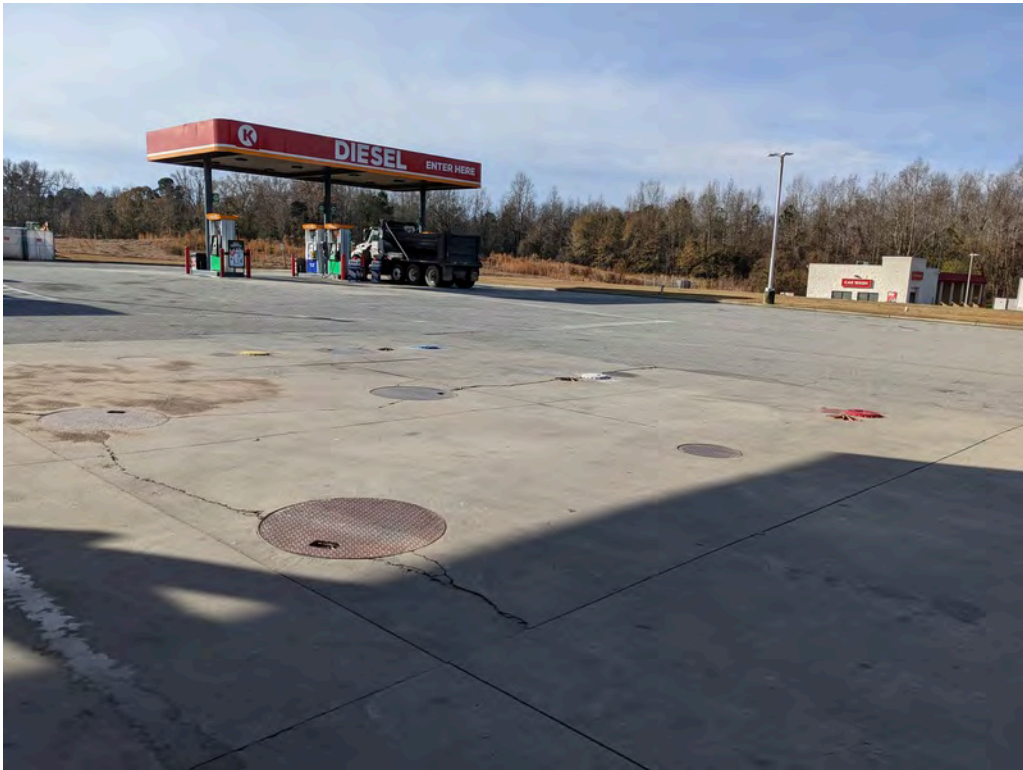
Northeast adjacent gas station tank pit located 80ft east of Subject Property
