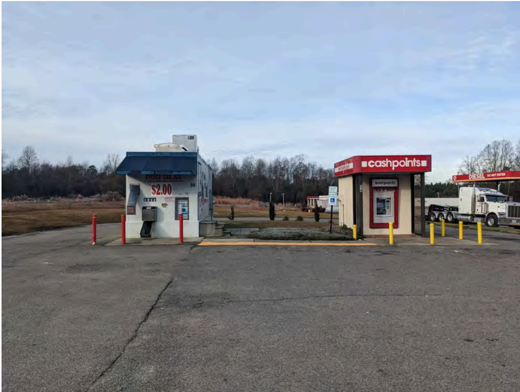
Subject Property Twice the Ice and Cashpoints ATM structures located on northeast portion of Subject Property
