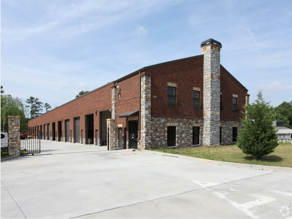
Building as seen from the street
