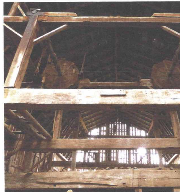
FIGURE 71 This odd renovation was perhaps done in the 1800s to gain precious mow space and install a wagon-rack-lifting wheel.
