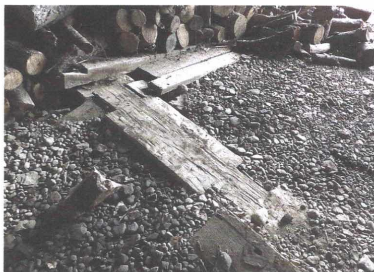
FIGURE 75 A 12 × 12 in. sill beam runs longitudinally the centre length of the barn, with 6 × 6 in sleeper beams transversely, 3 ft on centre.
