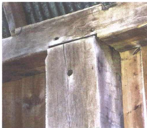
FIGURE 73 Hoisting pin holes were larger than pin holes in mortise-and-tenon joints because large pins were needed to withstand the stress of lifting heavy bents.
