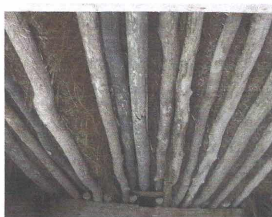
FIGURE 74 This crude mow of loose hay resting on the swing beam and beam of adjacent bent was likely built 70+ years ago, when loose hay was still common.
