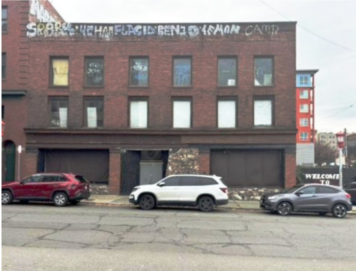
MAYNARD AVENUE SOUTH FRONTAGE, CLOSE VIEW
