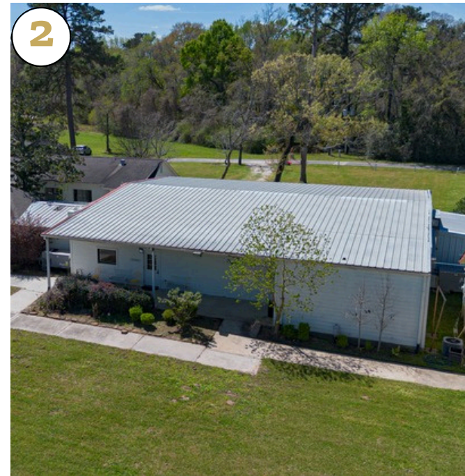
Building 2 Renovated: 2018 | 3,500 SF Event space with custom lights, commercial sprinkler system and bathrooms.
