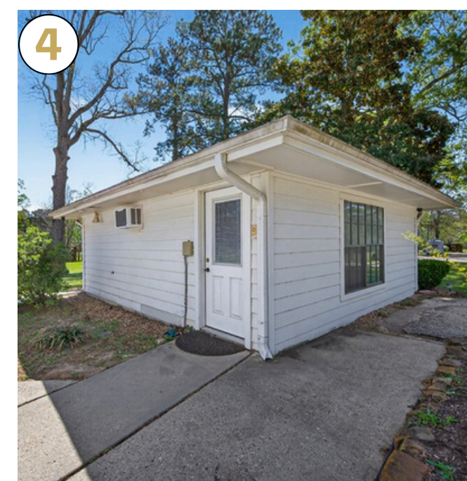
Building 4 404 SF Office or private room. Irrigation & Tech room.
