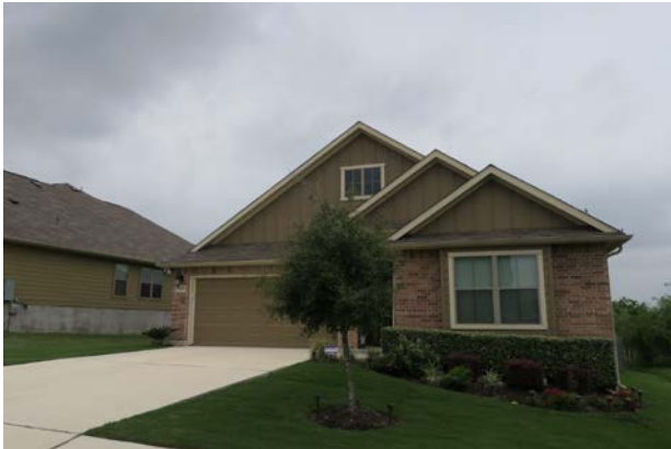
Southwest – typical single-family home in Cypress Point
