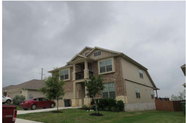
Southwest – typical single-family home in Cypress Point
