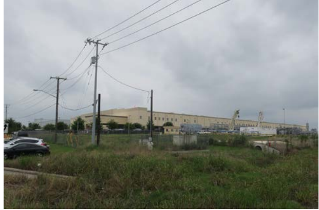
GE Oil & Gas facility
