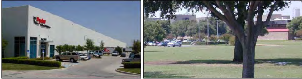
Images showing the desired character of development in the S5 Light and Heavy Industrial District (source: 2004 Comprehensive Plan Update, City of Pearland)
