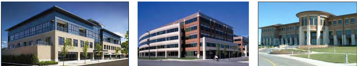
Images showing appropriate building materials within Research/Tech Campus Character Zone.
