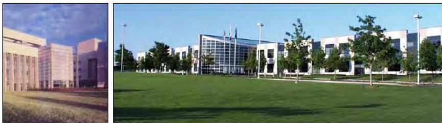
Images showing the desired character of development in the S4 Light Industrial and Science & Technology District (source: 2004 Comprehensive Plan Update, City of Pearland)
