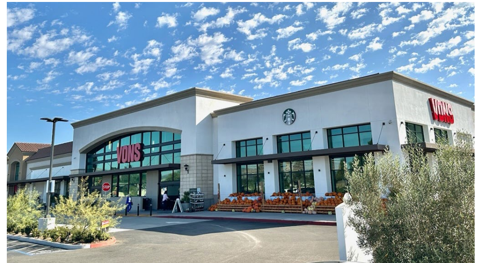
02 – Newly constructed 63,272 SF Vons
