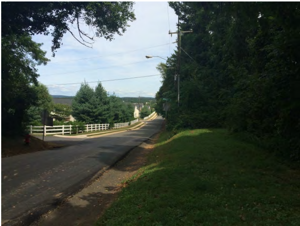
Photograph 4: View to the northeast showing Academy Hill Road located north of the subject site, and a power pole with a transformer, located along the northern site boundary.
