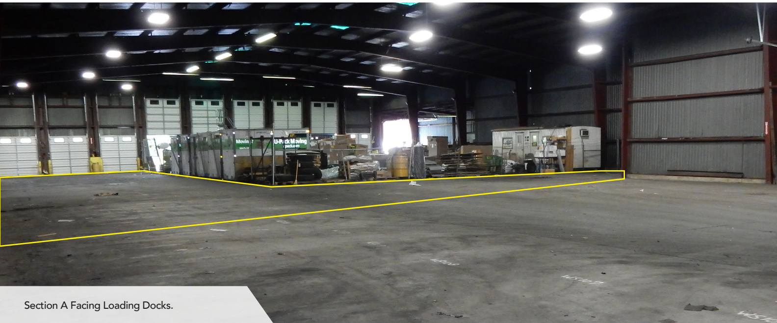
Section A Facing Loading Docks.
