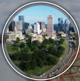
THE BORING COMPANY CONSTRUCTING A 13-MILE UNDERGROUND TRANSIT SYSTEM
