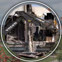
DEMOLITION BEGINS AT RIVERGATE MALL AHEAD OF $450M REDEVELOPMENT
