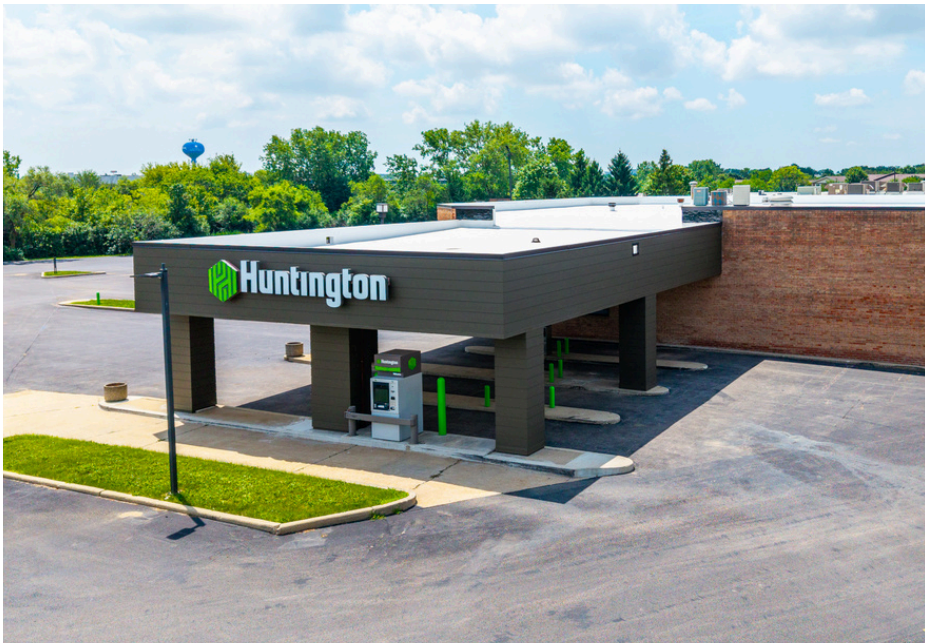
Newly constructed Bank Drive- Thru Canopy
