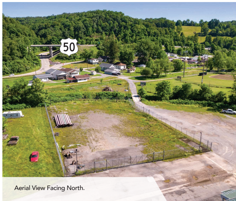
Aerial View Facing North.
