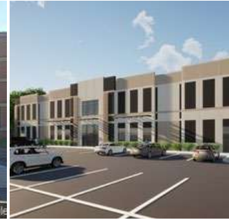
Highway 5 Business Center
