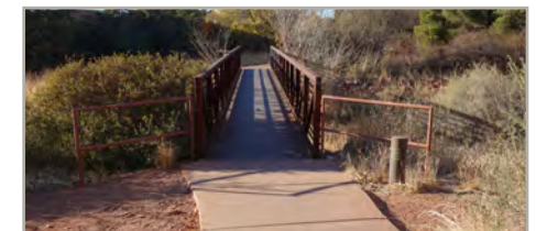
The Sunset Park pedestrian bridge over Carroll Canyon Wash
