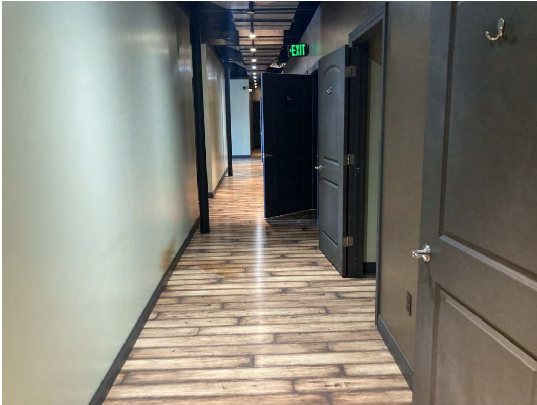
Photo 8: North portion of the building
