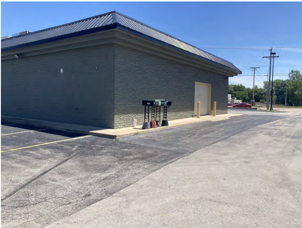
Photo 4: West side of the building facing south
