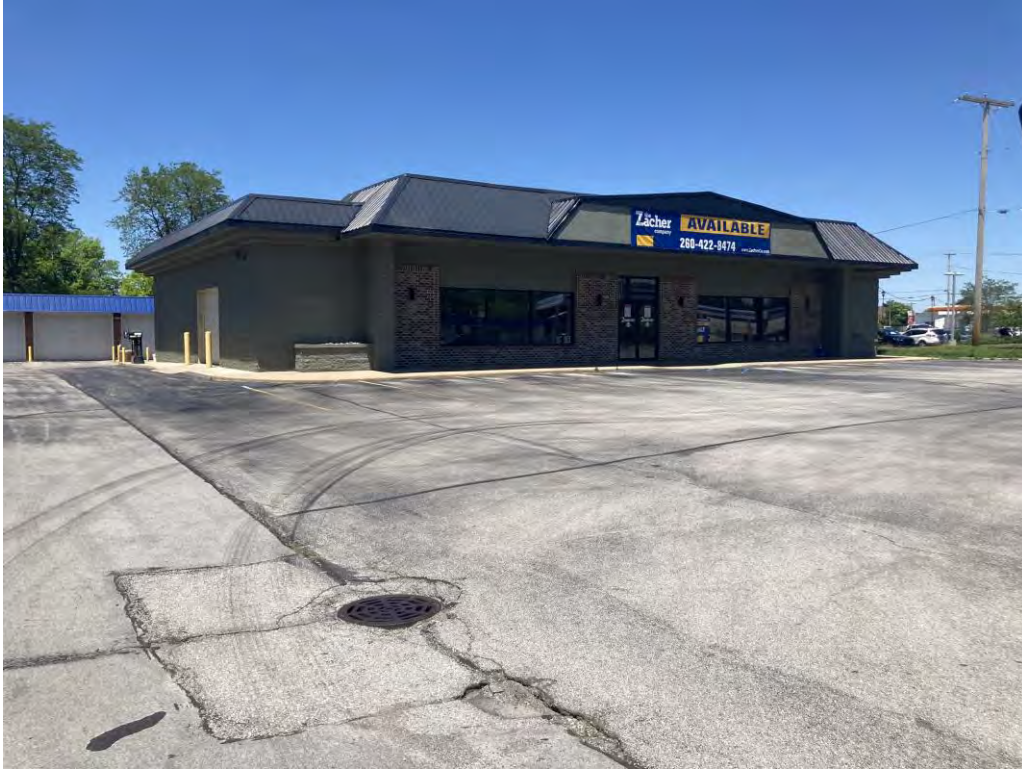
Photo 3: South and west sides of the building and south parking lot area facing north
