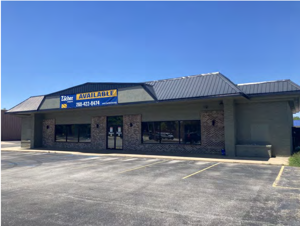
Photo 1: South side of the building facing north
