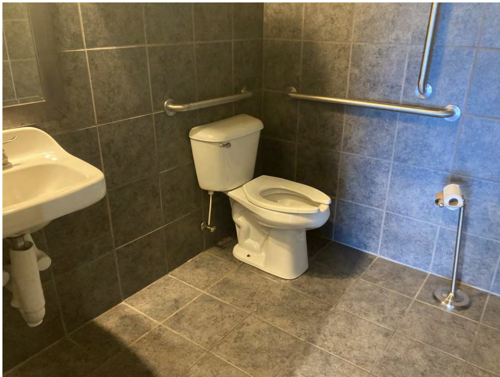
Photo 9: Restroom in the west portion
