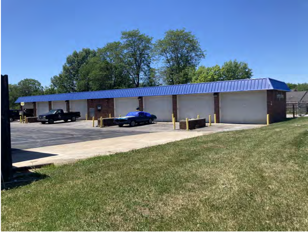
Photo 15: North adjoining former carwash building
