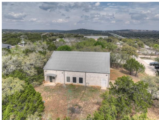
Aerial of back of office building
