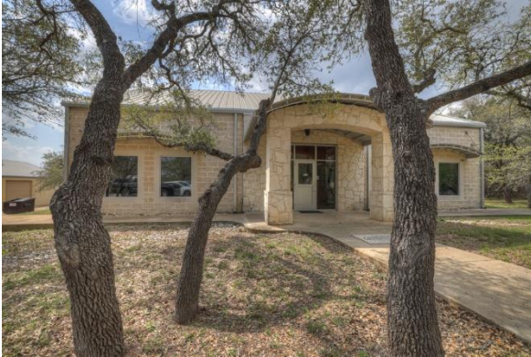
Office Building – Exterior Front
