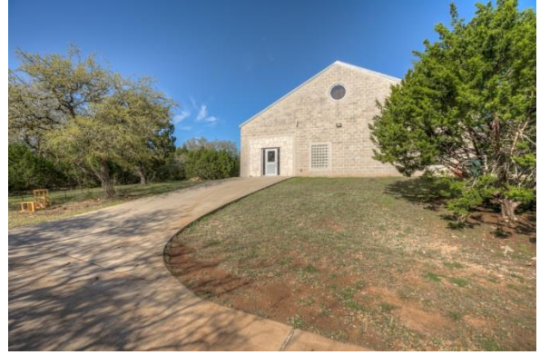
Office Building – Exterior Side
