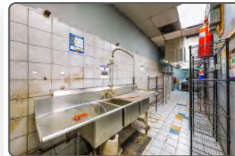
Kitchen Storage Area
