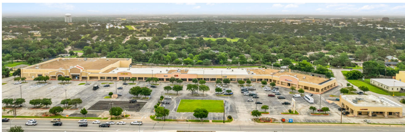
TOWNSHIRE SHOPPING CENTER
