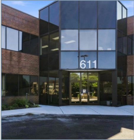
611 ENTRY - LOWER LEVEL UNITS
