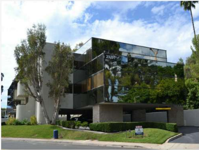
Building Photo (SW)
