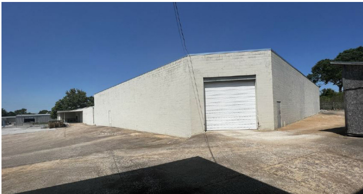
BUILDING ONE - 12' X 13' DRIVE-IN DOOR
