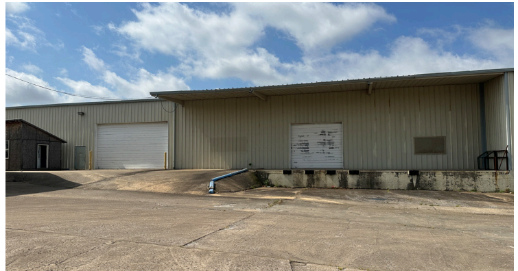
BUILDING TWO - COVERED 12' X 12' DOCK DOOR, 22' X 14' DRIVE-IN DOOR
