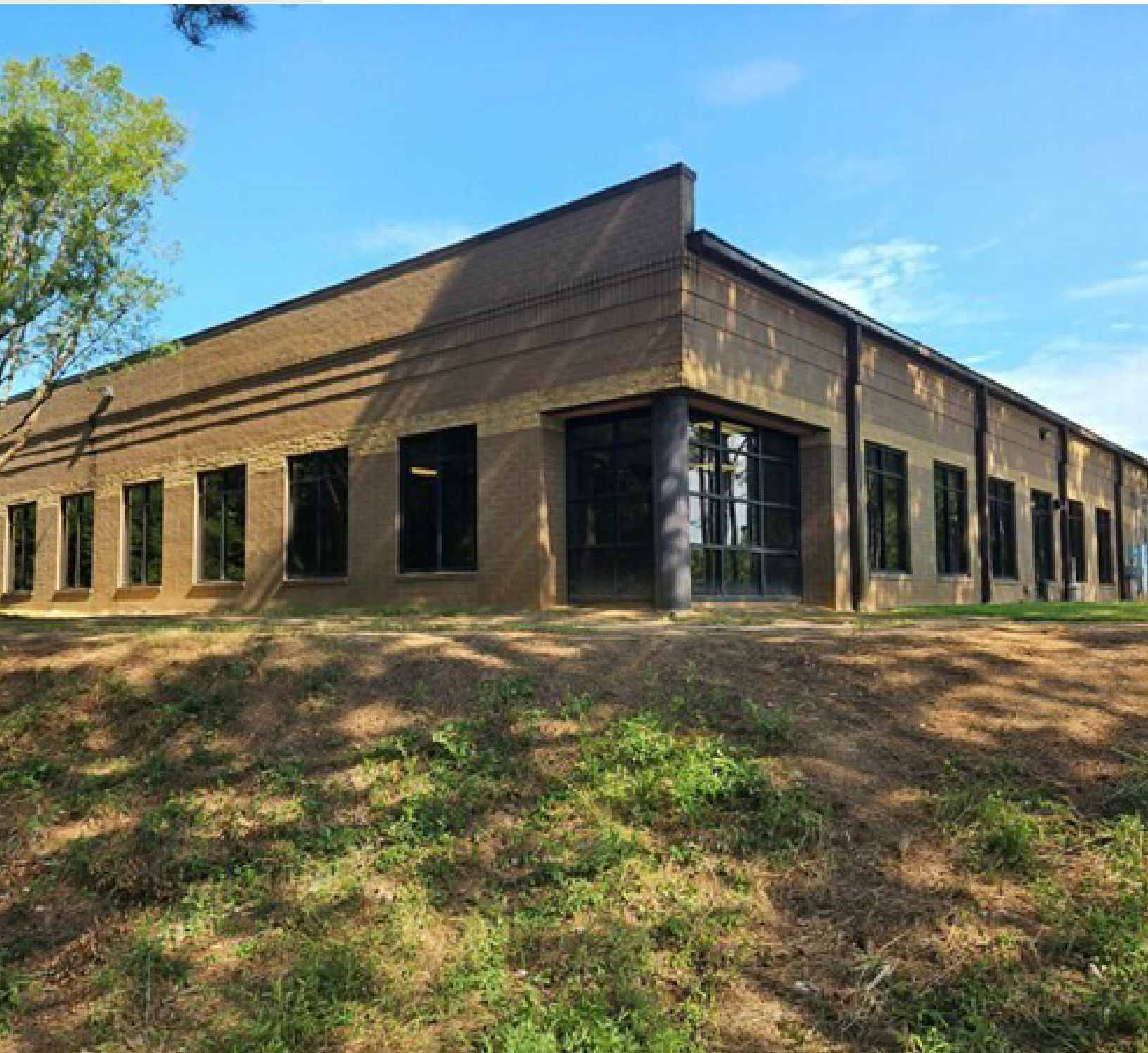
Back of Building
