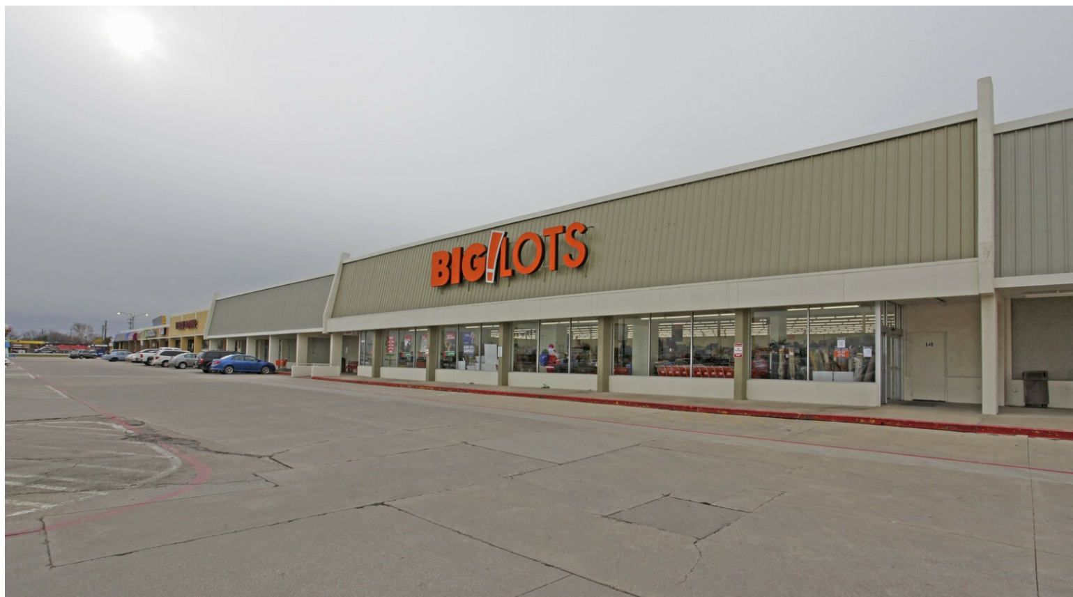
West Building Anchor
