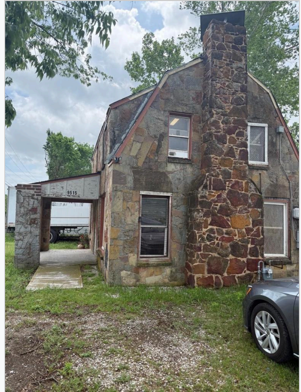
Office / Yard Access (9515)
