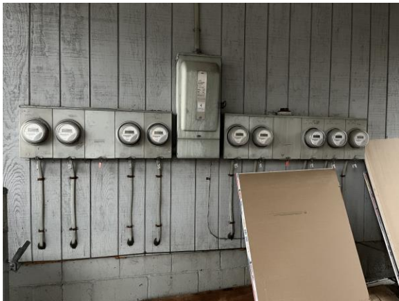
Electric Meters (8 residential unit meters and common area meter)
