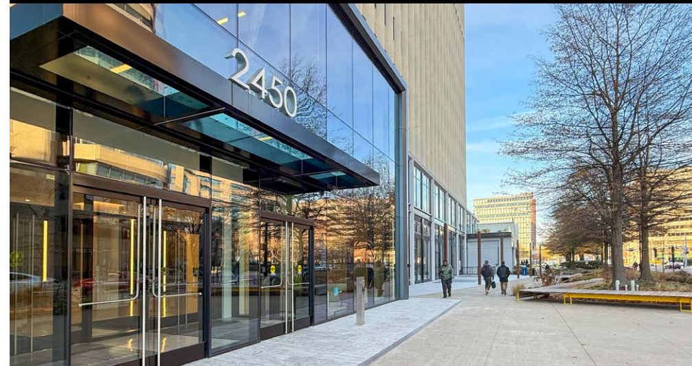
LOOKING NORTH ALONG THE CRYSTAL DRIVE STREETSCAPE
