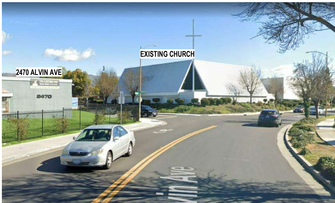
4) VIEW FROM ALVIN SHOWING EXISTING CHURCH
