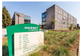
HORNET COMMONS Built in 2021, Hornet Commons is on-campus student housing with 284 apartments and 1,136 beds.
