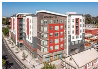
ACADEMY 65 Built in 2019, Academy 65 is off-campus student housing with 90 apartments and 300 beds.
