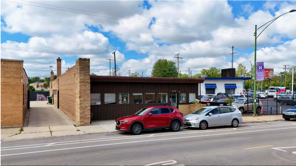
Front - North East - Elevation
