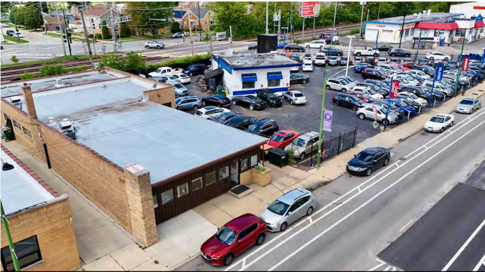
Northeast Elevation - Proximity to Nagle
