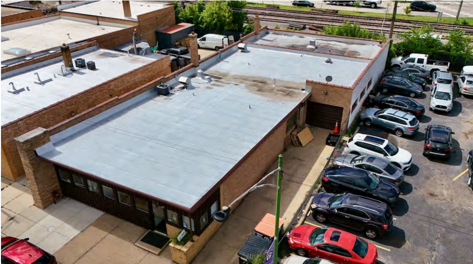
Northwest Elevation - Driveway and Drive-in Door
