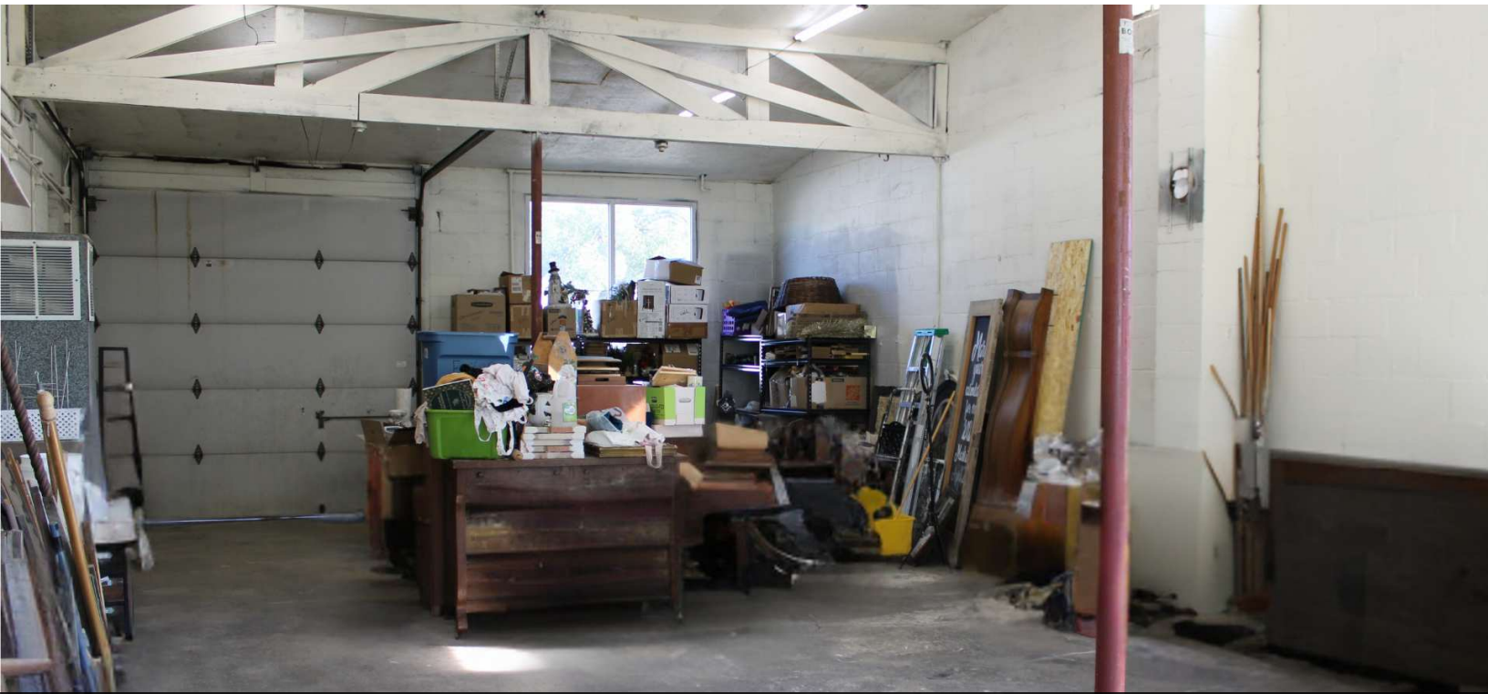
1126 sf of Shop/Storage Space with Overhead Door
