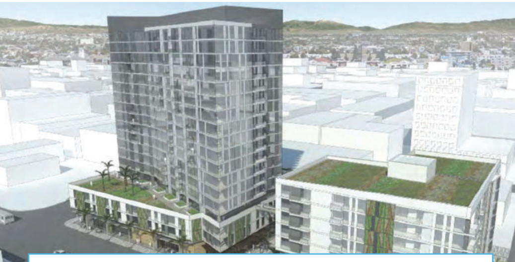
This ambitious zz near the Pacific Avenue Blue Line station would replace a parking lot with a pair of residential structures with 325 units, according to a recent presentation from Mayor Robert Garcia.
