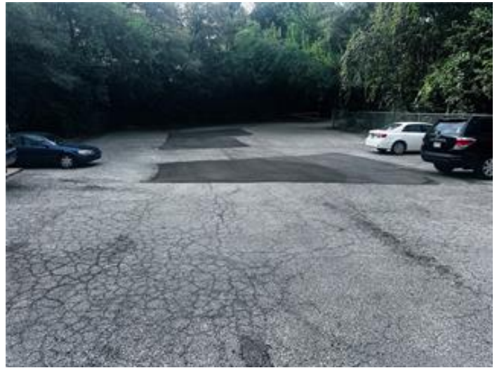
rear outside storage area
