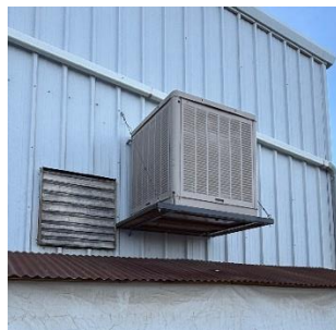
Evaporative Cooler in Main Shop
