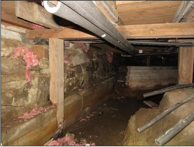
5.4 Item 1(Picture) Crawlspace
