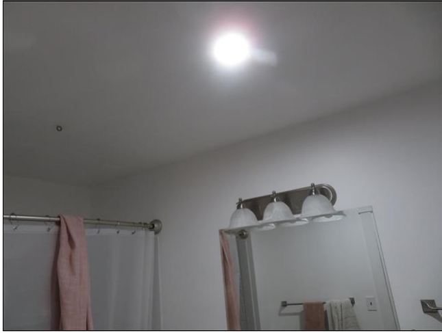
4.19.B Item 1(Picture) Bathroom
