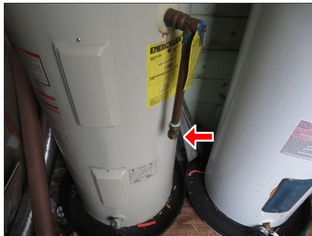
4.10.B Item 2(Picture) Utility room
