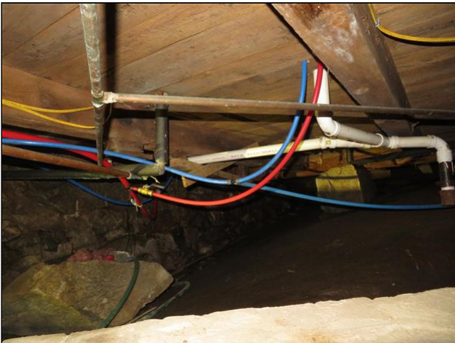
6.1 Item 1(Picture) Crawlspace
