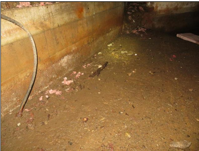
5.1 Item 6(Picture) Basement
