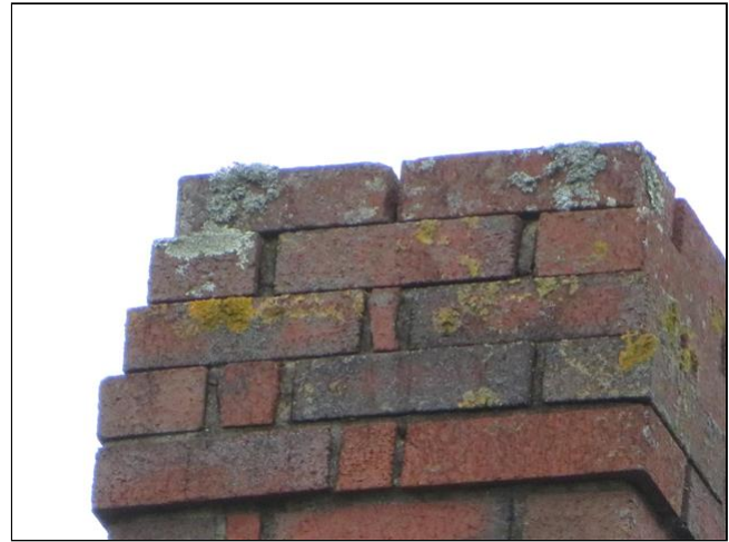
2.3 Item 6(Picture) Left side chimney
