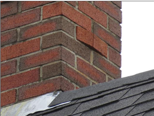
2.3 Item 9(Picture) Left side chimney
