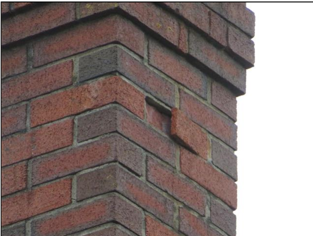
2.3 Item 7(Picture) Left side chimney
