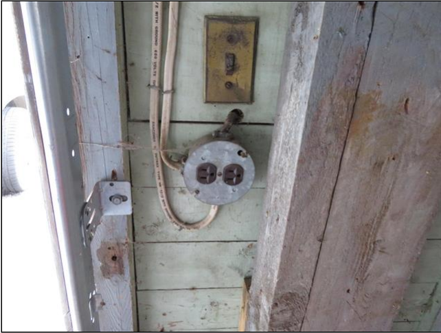
7.4 Item 1(Picture) Attached garage
