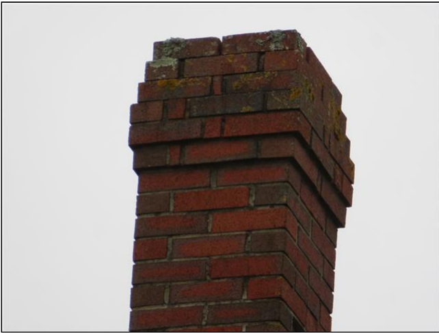
2.3 Item 5(Picture) Left side chimney
