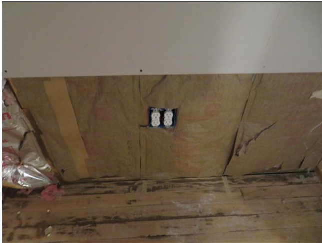
4.15.A Item 2(Picture) Utility room
