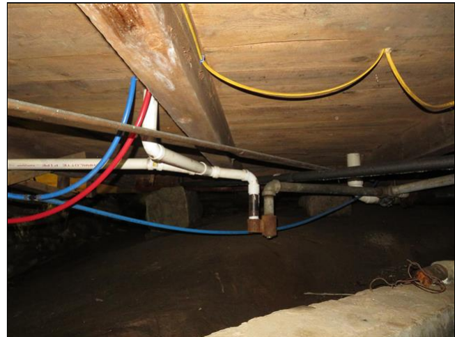
6.1 Item 2(Picture) Crawlspace
