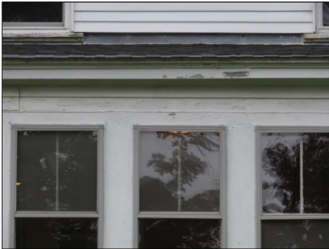
1.7 Item 3(Picture) Front
