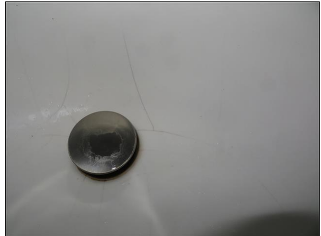
4.8.A Item 2(Picture) Hall bath
