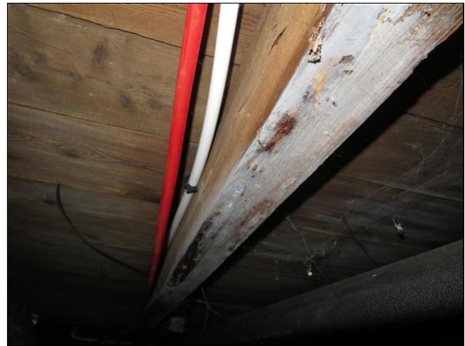
5.5 Item 2(Picture) Crawlspace
