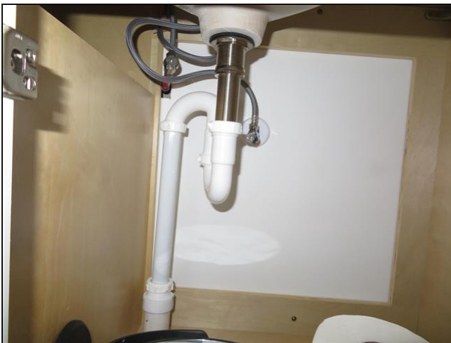
4.8.B Item 1(Picture) Bathroom
