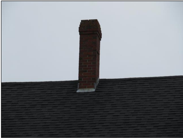
2.3 Item 1(Picture) Left side chimney
