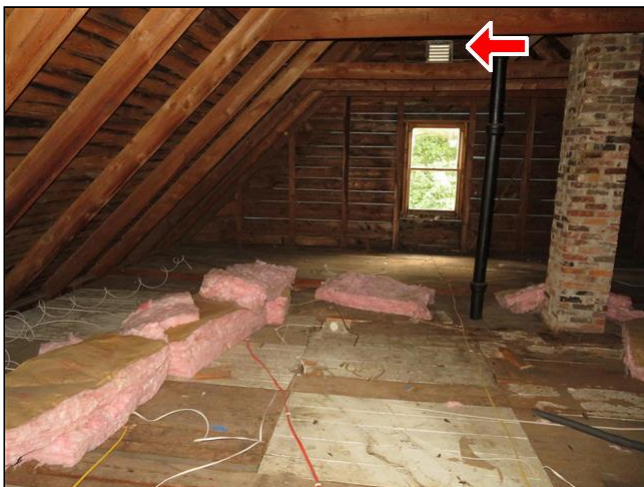
9.3 Item 1(Picture) Attic
