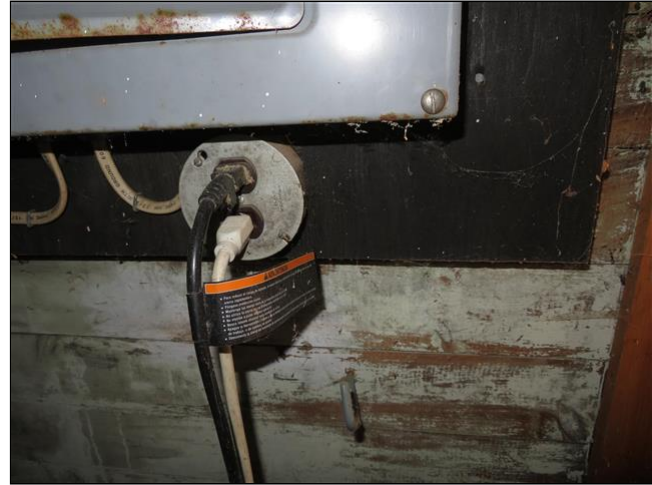
7.4 Item 2(Picture) Attached garage
