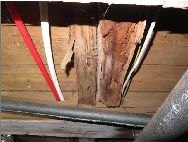
5.5 Item 1(Picture) Crawlspace
