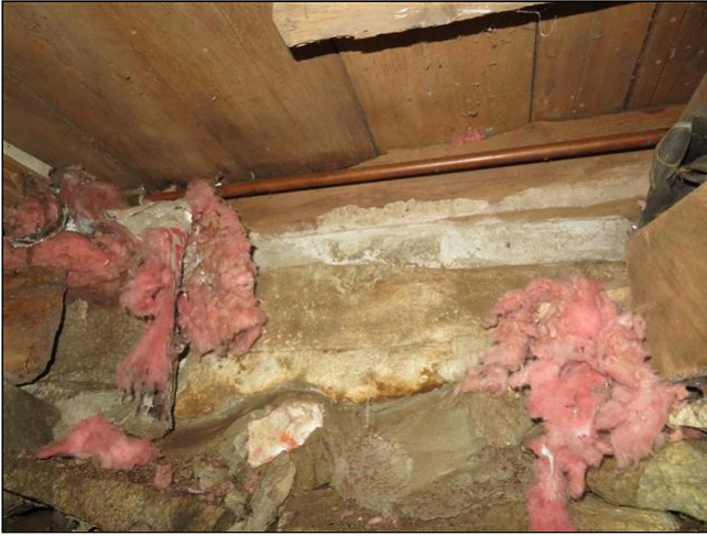
5.1 Item 7(Picture) Basement
