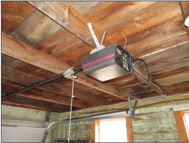
3.8 Item 1(Picture) Attached garage
