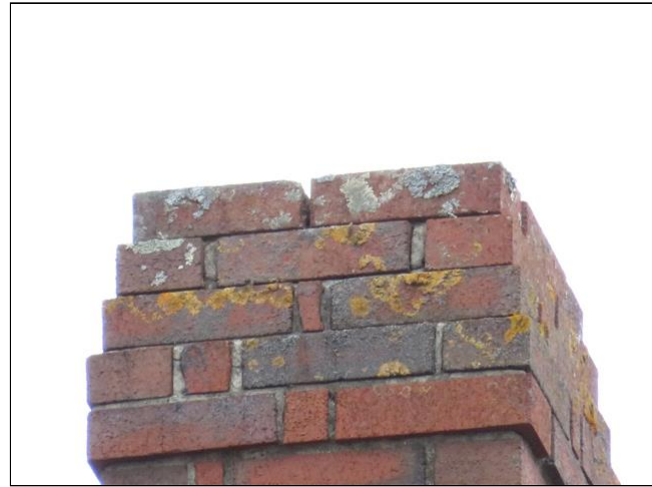
2.3 Item 2(Picture) Left side chimney
