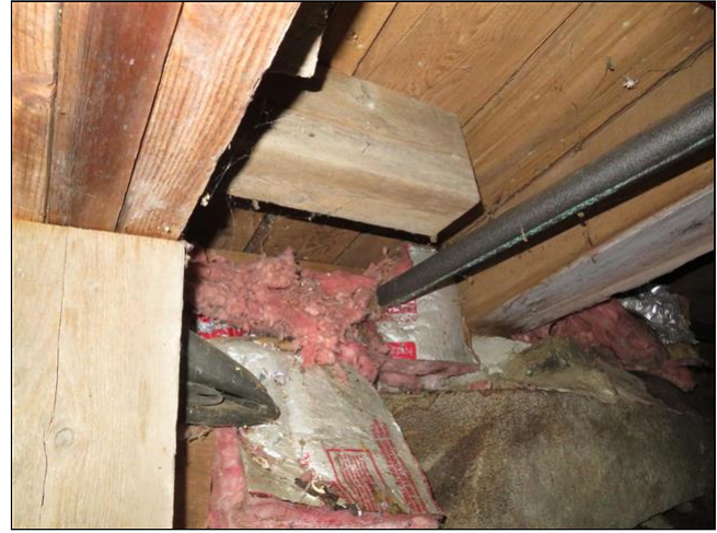
5.1 Item 8(Picture) Basement
