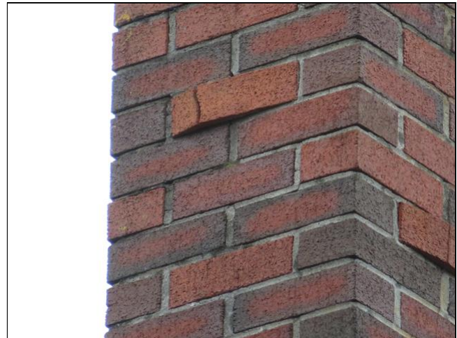
2.3 Item 8(Picture) Left side chimney
