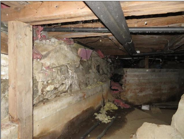
5.1 Item 3(Picture) Crawlspace
