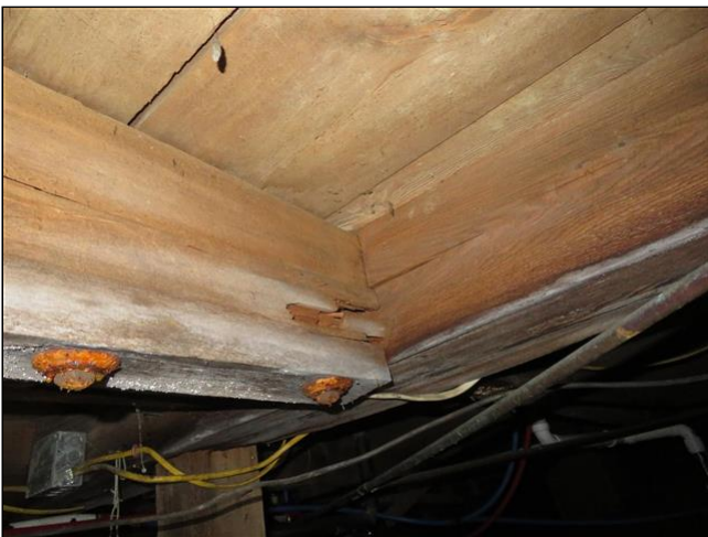
5.5 Item 3(Picture) Crawlspace
