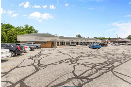
Front of Structure
