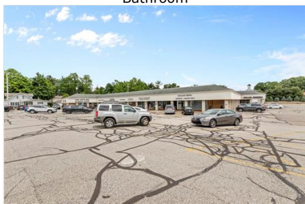
Front of Structure
