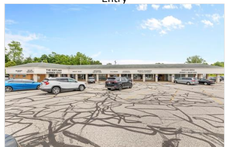
Front of Structure
