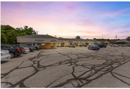
Front of Structure
