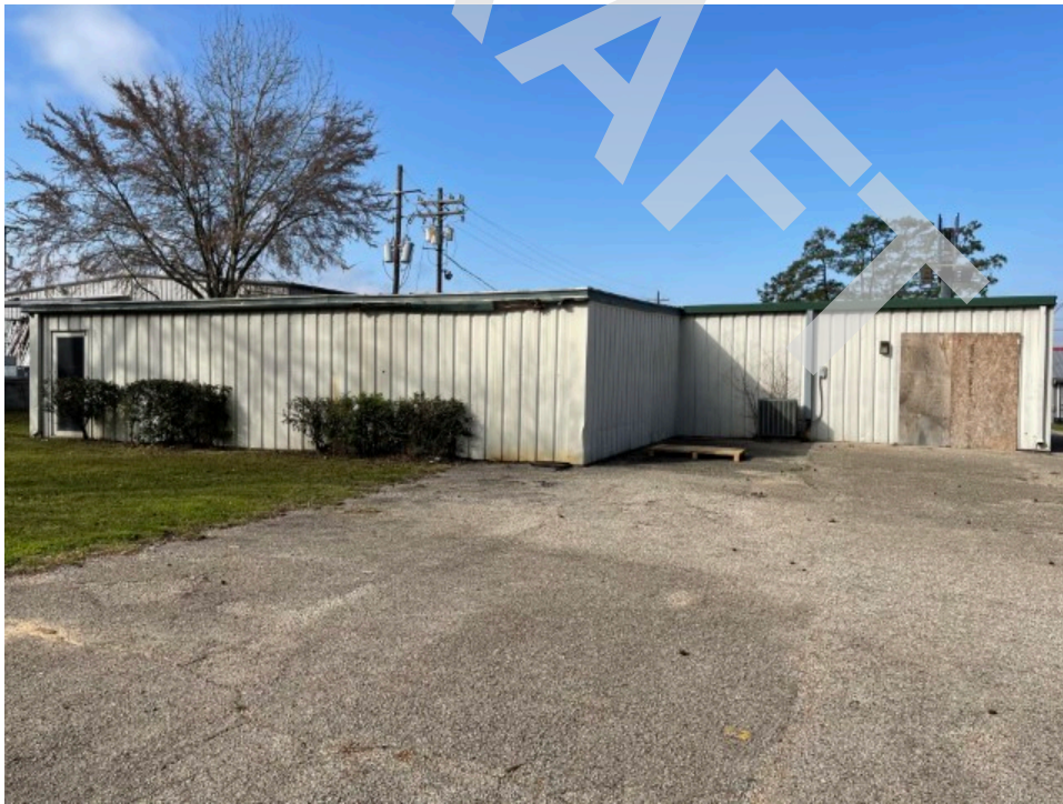
6. Rear or east side of office building
