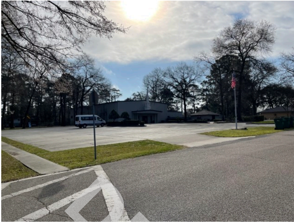
21. Adjoining property to the east
