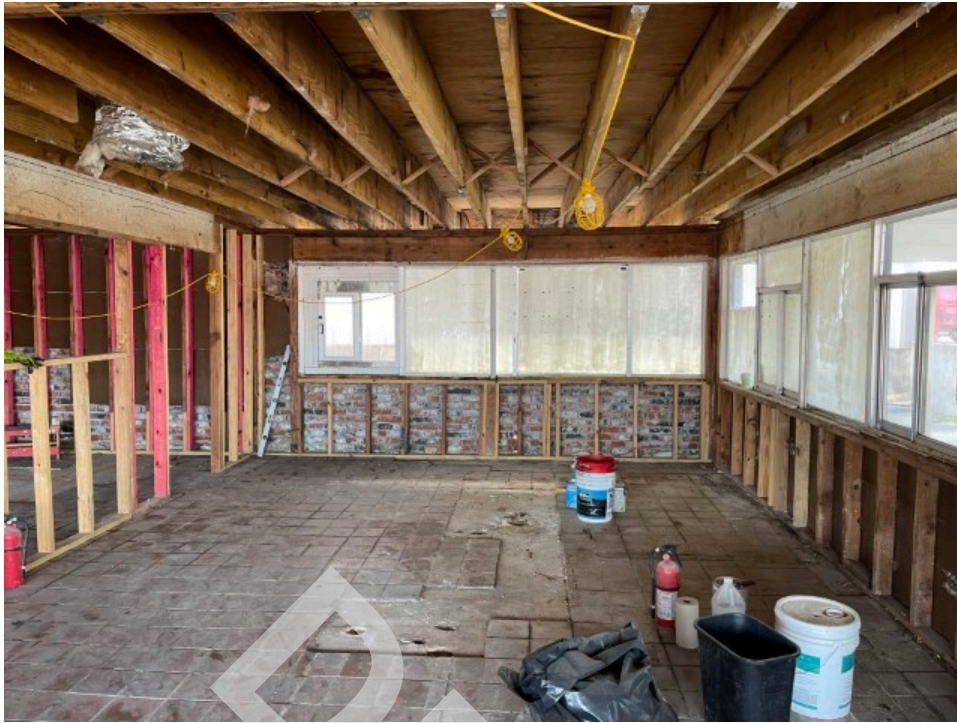
7. Interior of former Dairy Queen building
