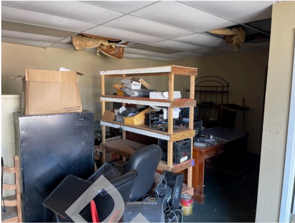
9. Interior of office building
