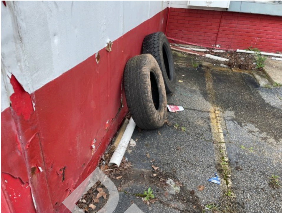
15. Old tires observed on subject property
