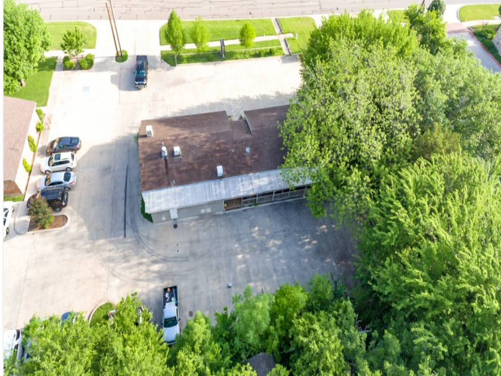
Exterior overhead rear, close
