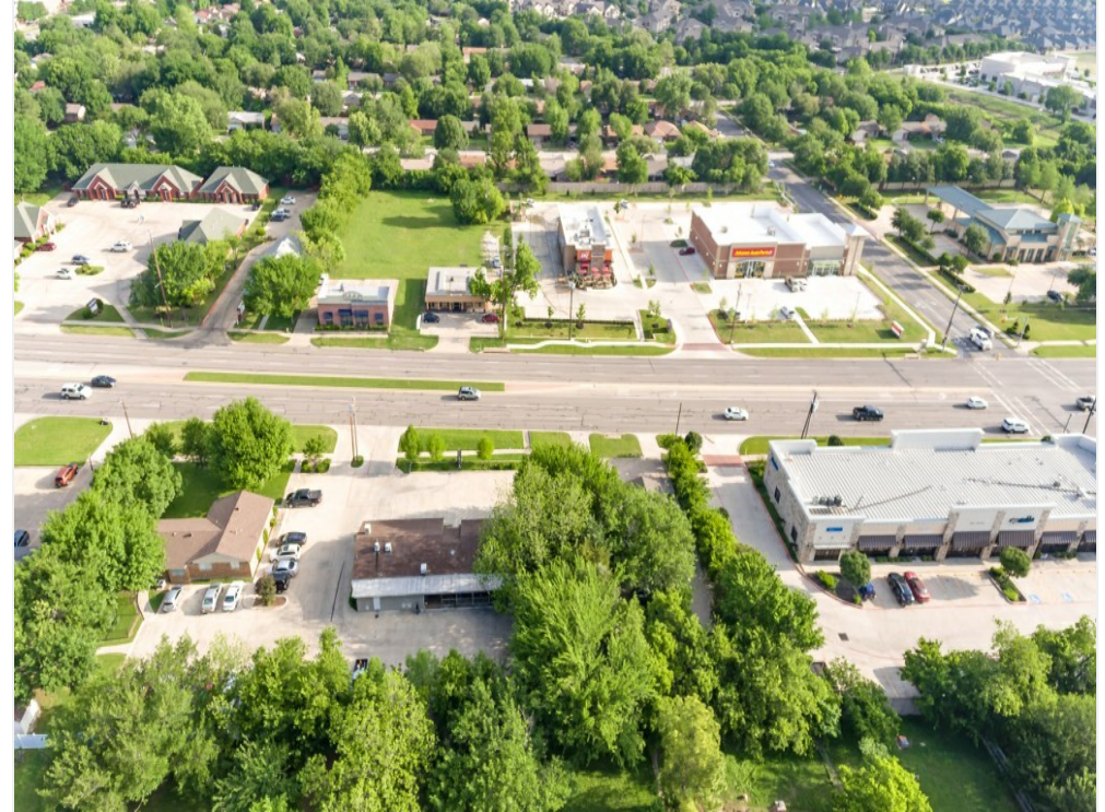
Exterior overhead rear, far
