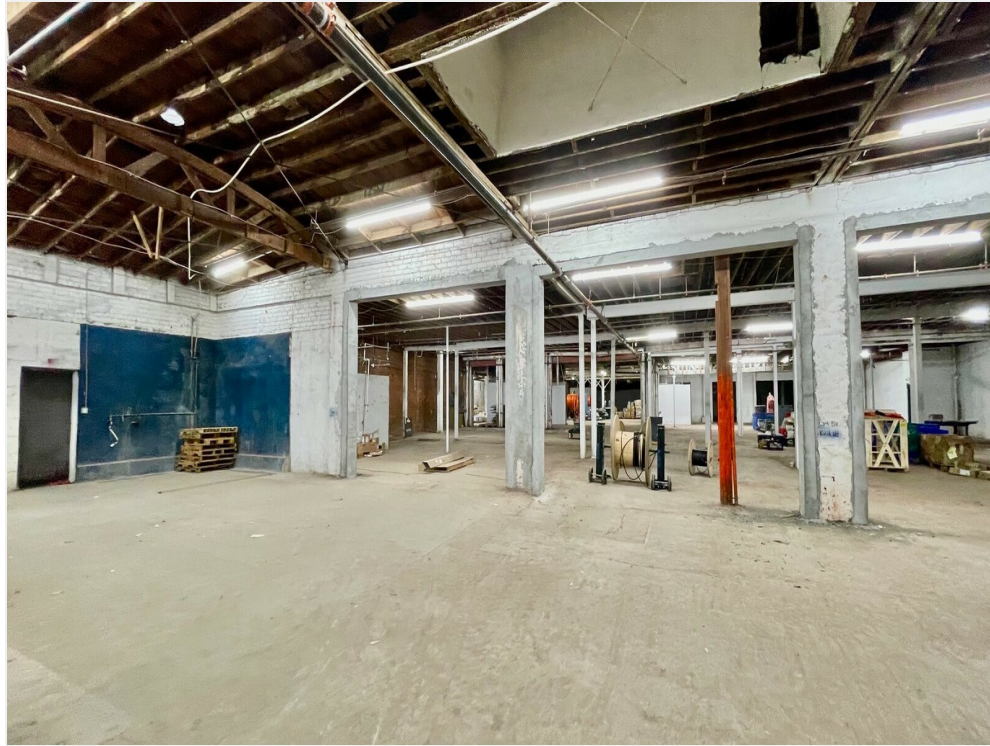
Interior photo 2200 89 St
