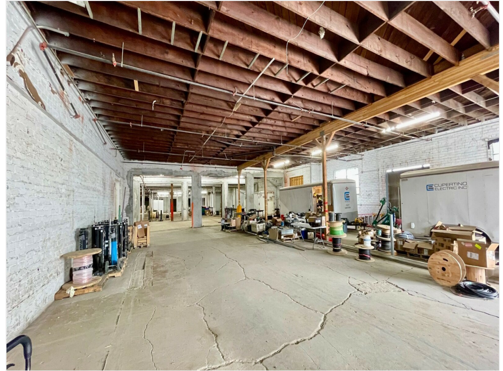
interior photo 2200 89 St
