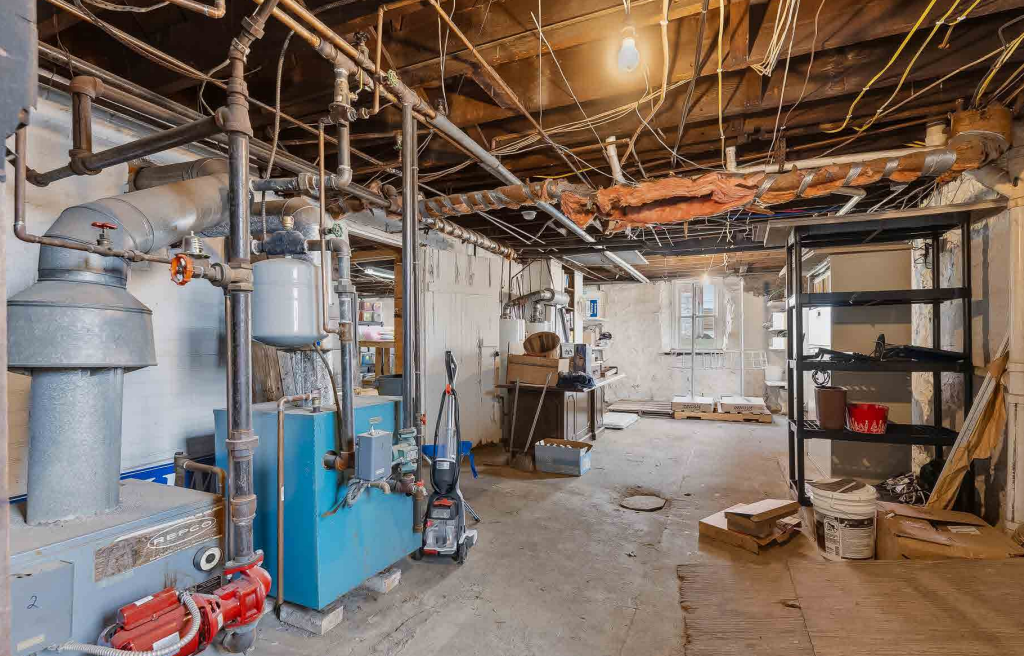
Main Building Basement.
