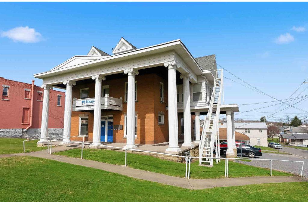
Exterior View from Morgantown Ave.
