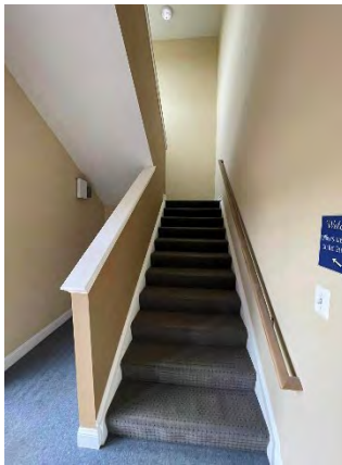
One of Two Stairwells
