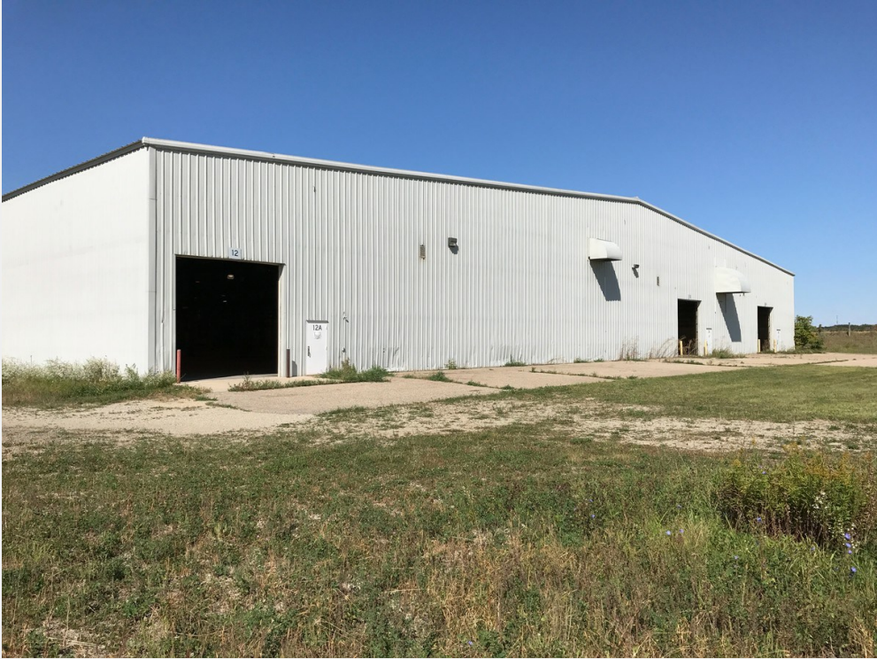
Mfg Section of Bldg - Rear view
