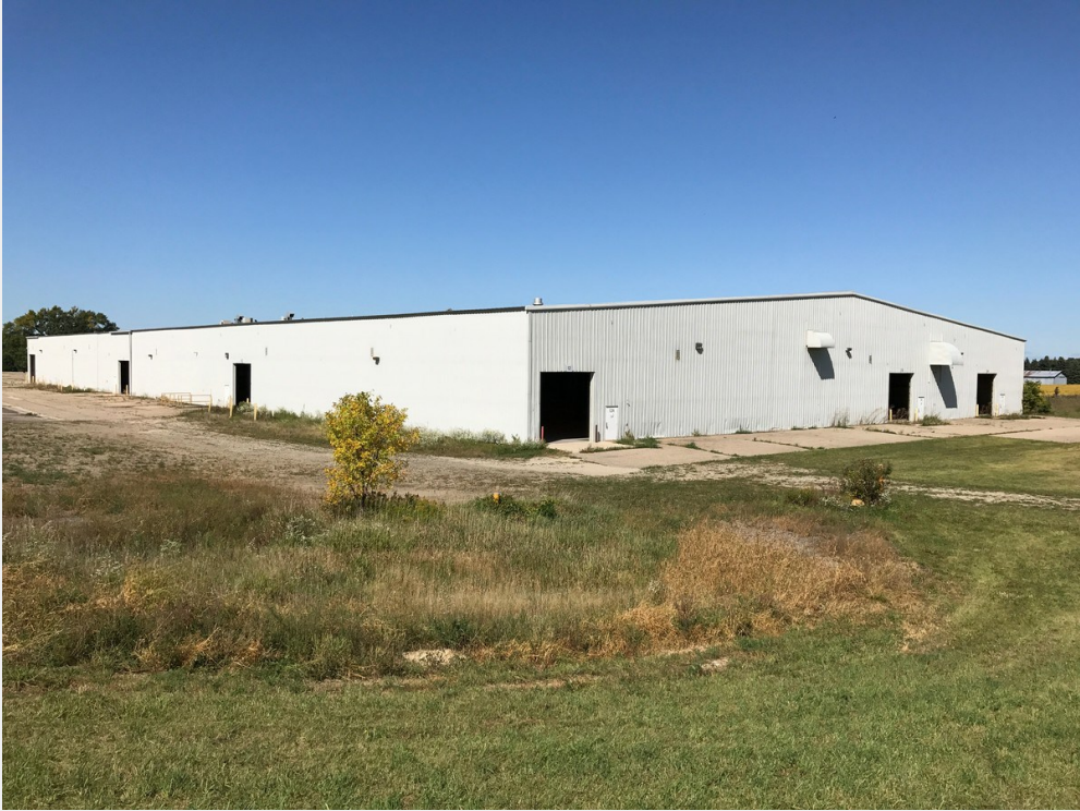
Mfg Section of Bldg - Rear overall view
