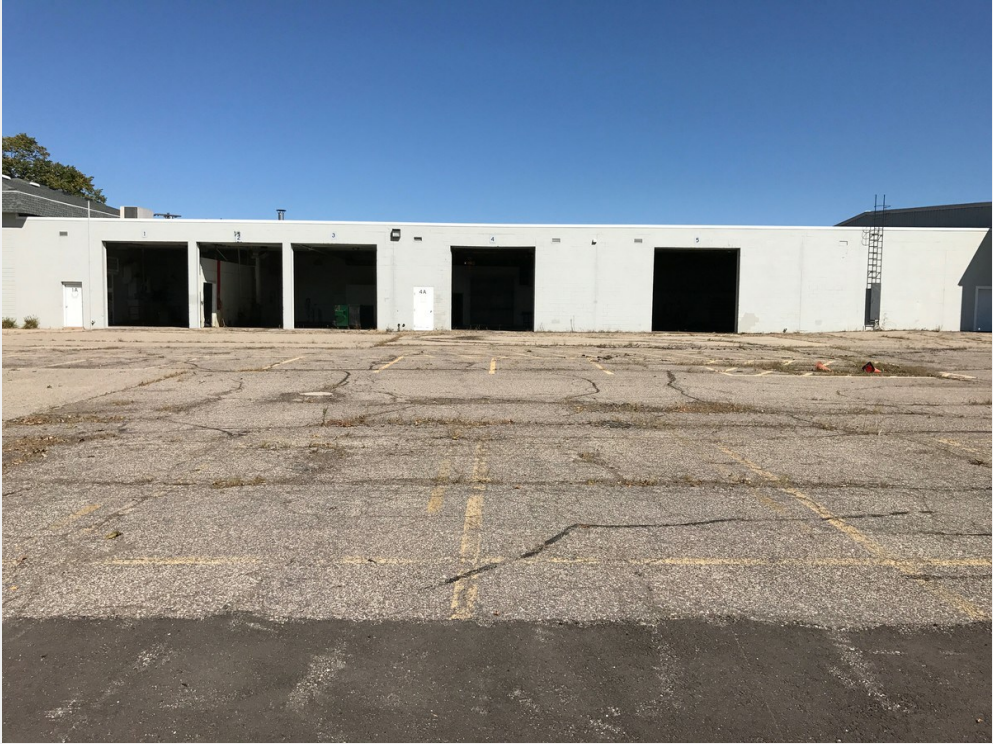
R & D Section of building with 5 drive-in doors and several overhead cranes
