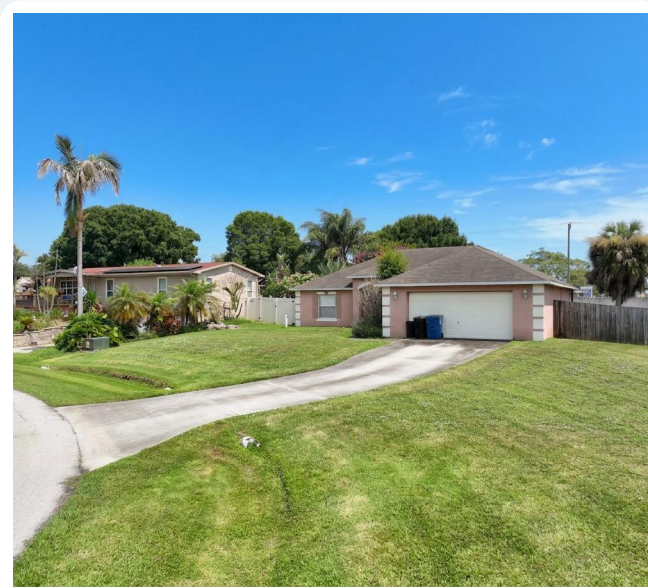
CORNER RESIDENTIAL IMPROVEMENT
