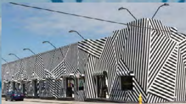
WYNWOOD BUILDING Goldman Properties 45,000 SF
