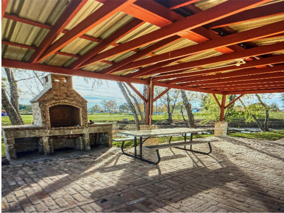
Outside Kitchen and Fireplace
