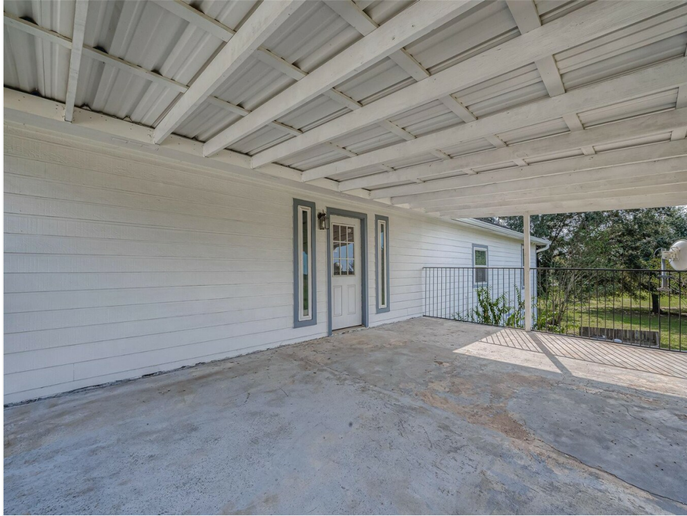
Front Covered Porch
