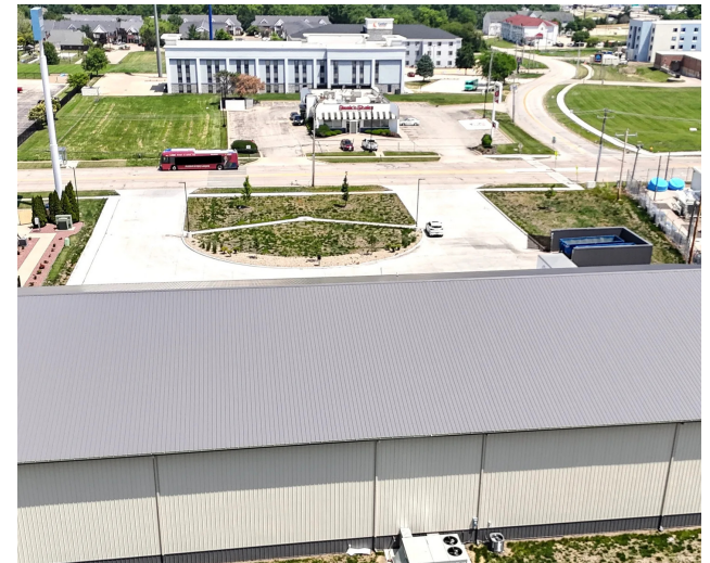
Back side of property
