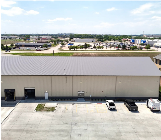
Front entrance, two docks and one drive-in
